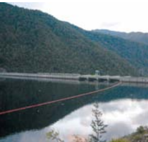
Pangué Hydroelectric power plant, Chile
