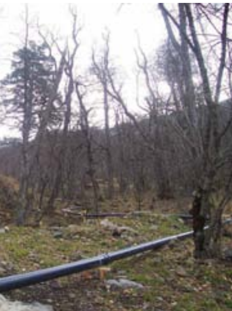
Water pipe installed after CAO process, Tsemi, Georgia
