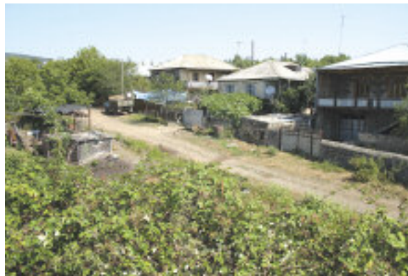
CAO helped to resolve complaints from a number of Tetrtskaro residents in Georgia who believed that the BTC Pipeline Co. was responsible for cracked walls in their homes.
