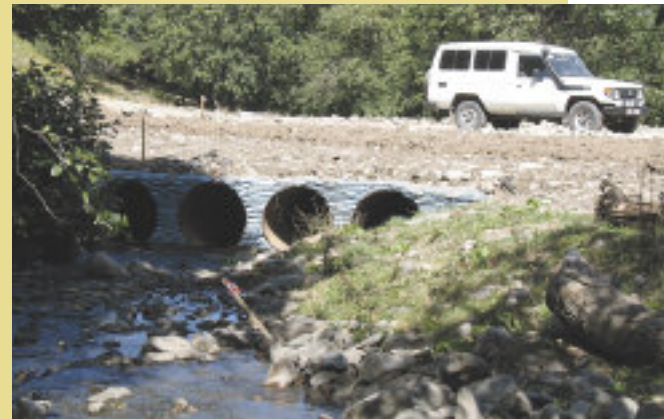
As part of a settlement facilitated by the CAO Ombudsman in 2006, BTC Pipeline Co. agreed to install a new water pipe for residents of Tsemi Village in Georgia.
