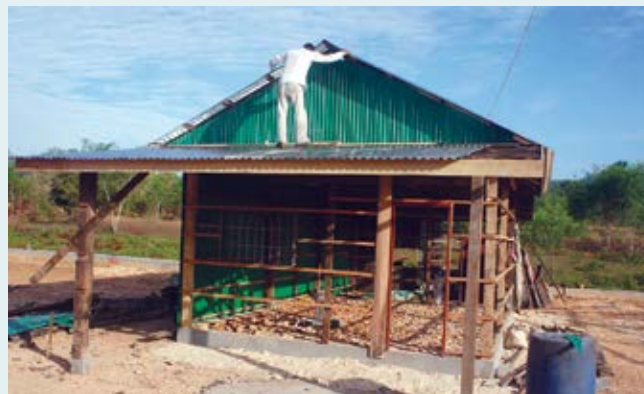
New home under construction for a resettled family near Sihanoukville, Cambodia.
