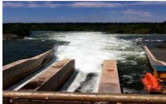
The Bujagali power plant
