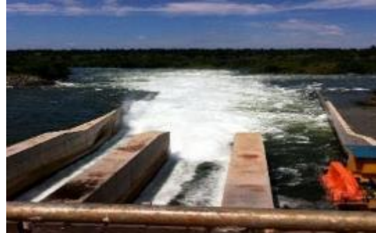
The Bujagali power plant
