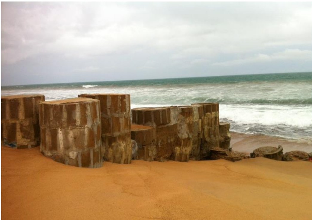
Exemple of protection work constructed by the communities in Kossi Agbavi
