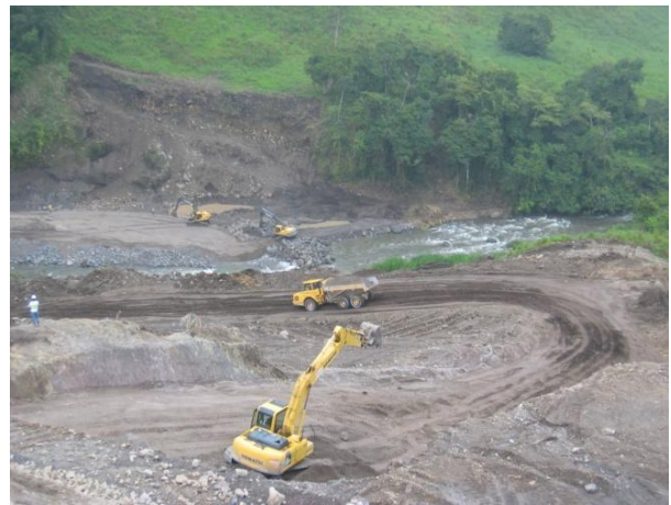
EISA hydroelectric plant construction, Chiriquí Viejo River, Panama
